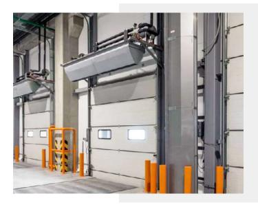
Air curtains are equipment that **creates an invisible air barrier in the interior and the outside of a chamber**, maintaining the thermal conditions in it and allowing the passage of people or vehicles.
