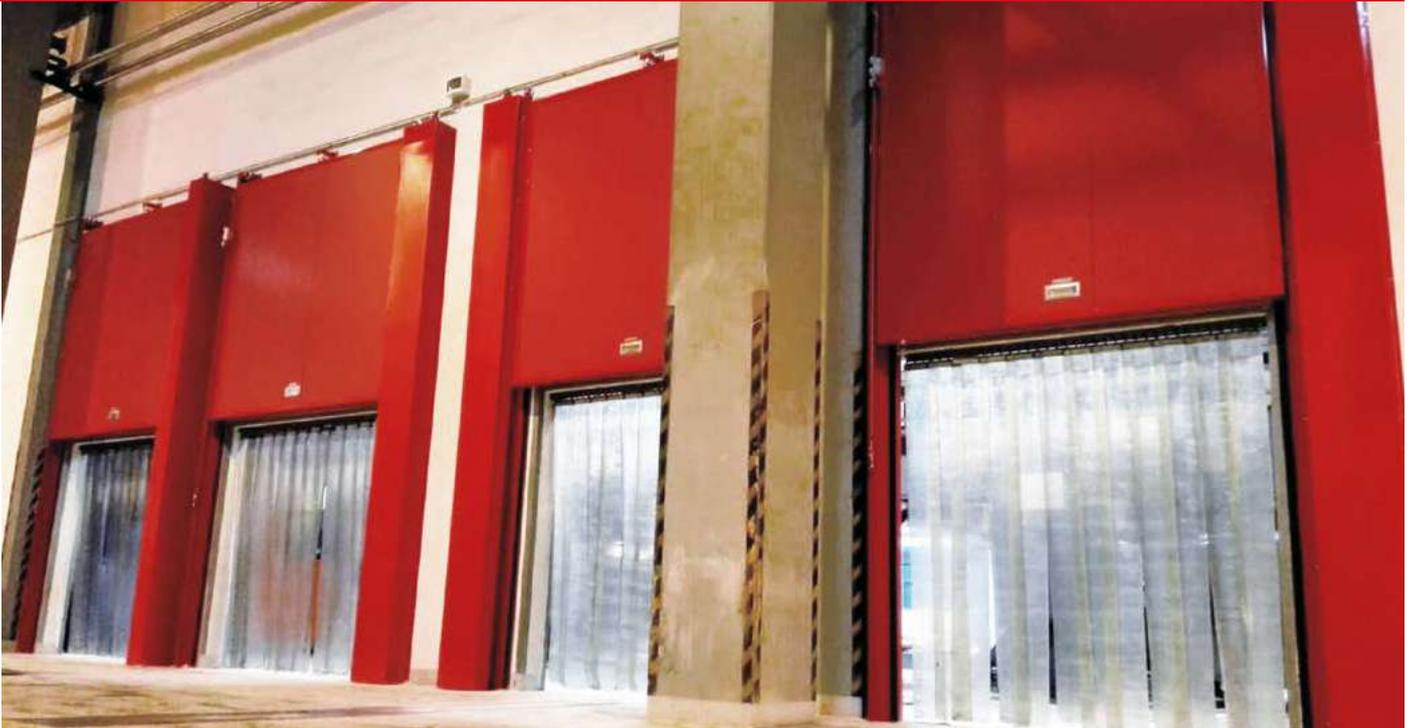
Kavidoors fire guillotine doors are designed for **access areas where there is no lateral clearance but there is free height**. They **resist fire for one hour**. They usually remain open, **held by an electromagnet**, until, in the event of fire detection or a power failure, the counterweight system causes the **doors to close automatically**.
